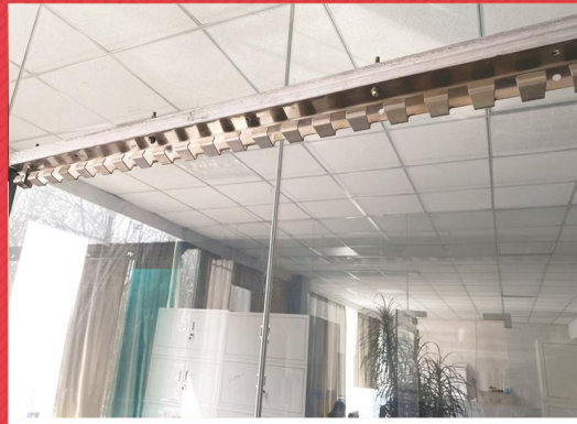
② Fix the keel with screws
